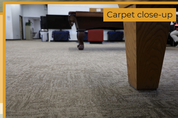
New floor in office
